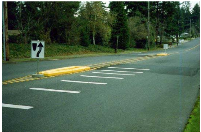
Split Speed Hump Source: City of Portland, Oregon
